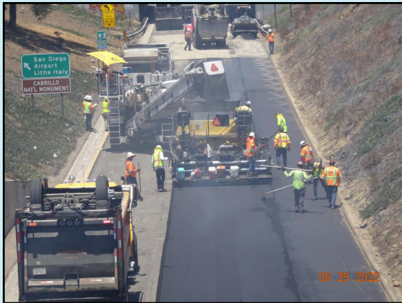
Placement of HyRAP® Hot Mix Asphalt
