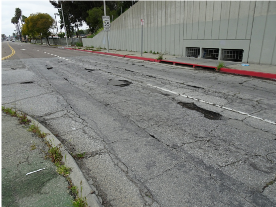
POTHOLING CAUSED BY RECENT RAIN EVENTS
