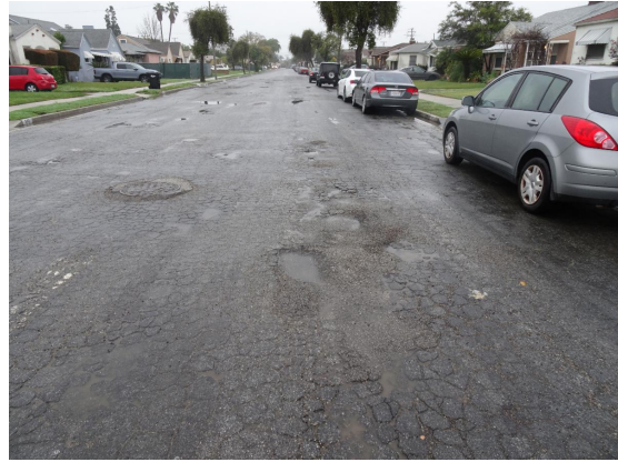
POTHOLING CAUSED BY RECENT RAIN EVENTS
