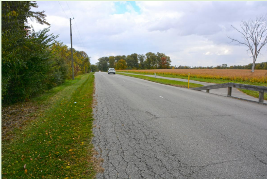
Current Condition of Conventional HMA Control Section Placed October, 2012.
