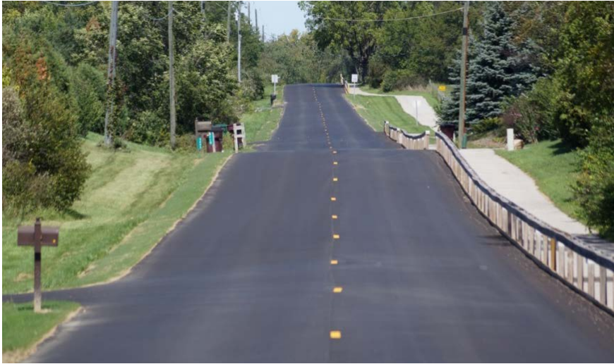
Fig. 4 Eggeman Road, Fort Wayne, Indiana – shortly after construction with overly containing 100% recycled asphalt
